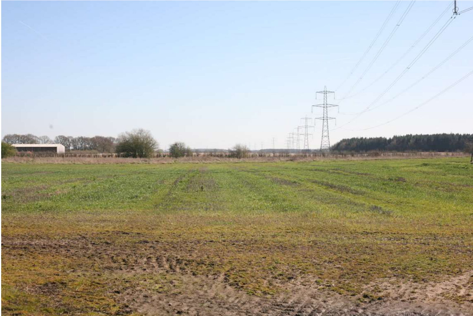
Photograph looking south across the site showing overhead lines
